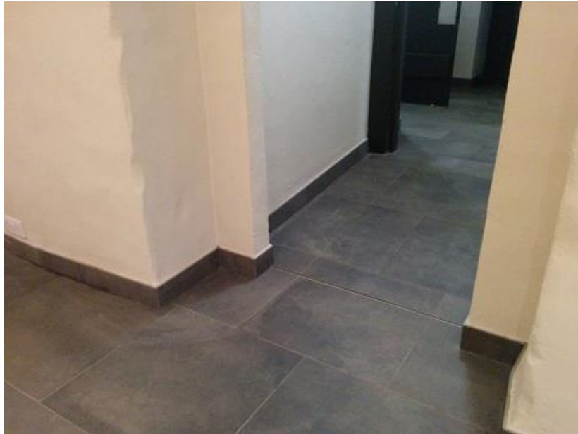
Photo 23: The slight level change to reach the toilets
