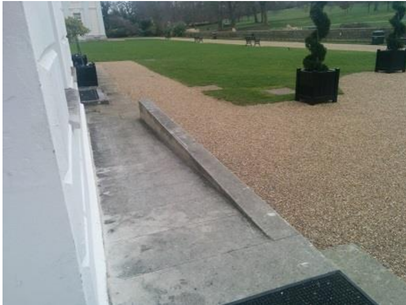
Photo 16: The external ramp to the Orangery from the South side of the House
