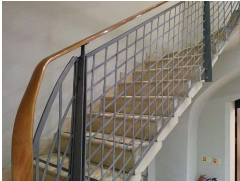
Photo 8: The West Staircase
