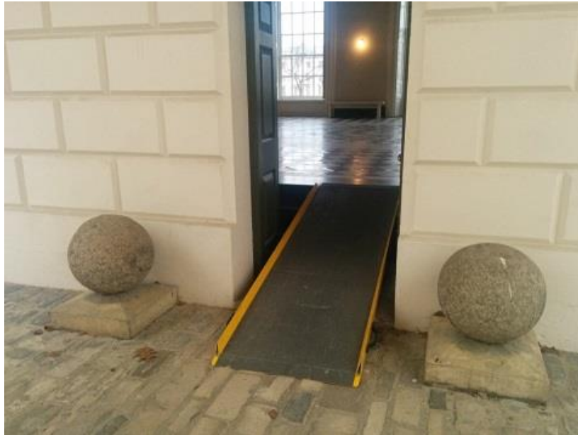
Photo 18: The portable ramp set up from the Great Hall to the carriageway
